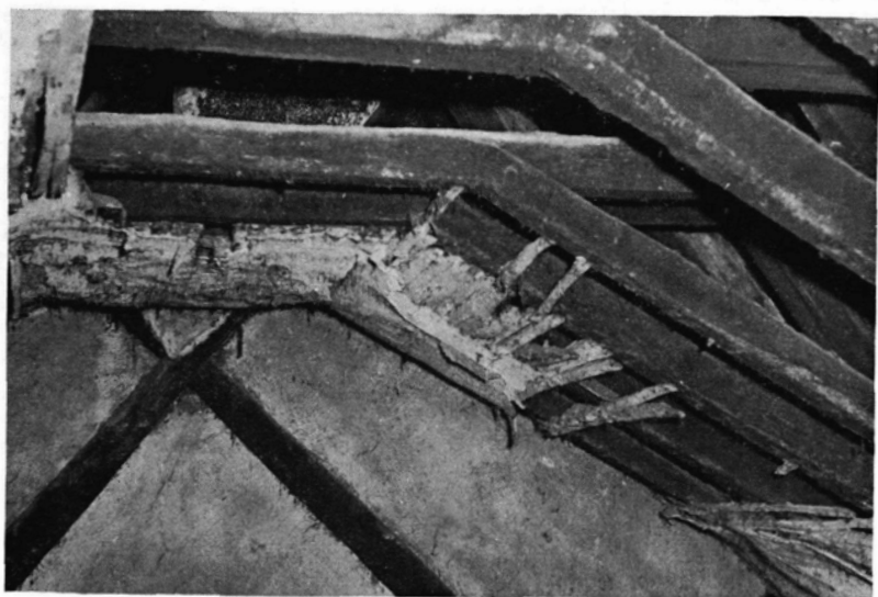
A. The Hall Roof.
